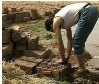
Fig2 General view of molding Mud brick, Source: [10]
