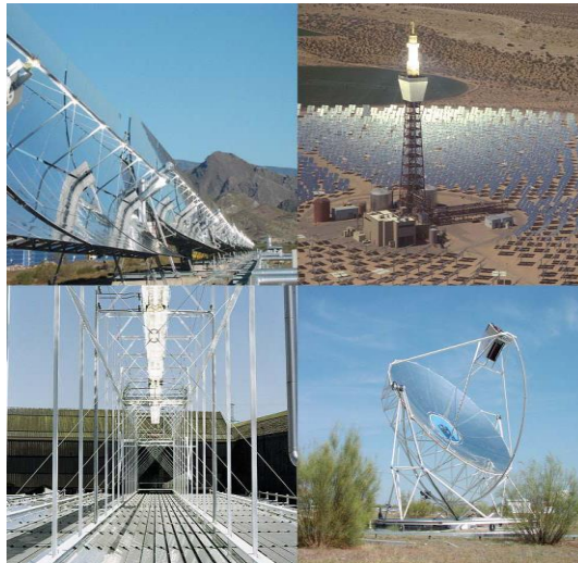
Figure 2. Four mainstream CSP-technologies.
