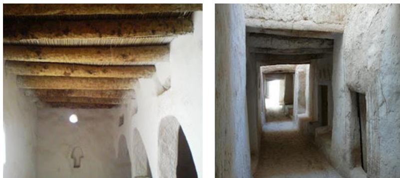
Fig3 Using palm trunks in ceiling, Source: [10].
